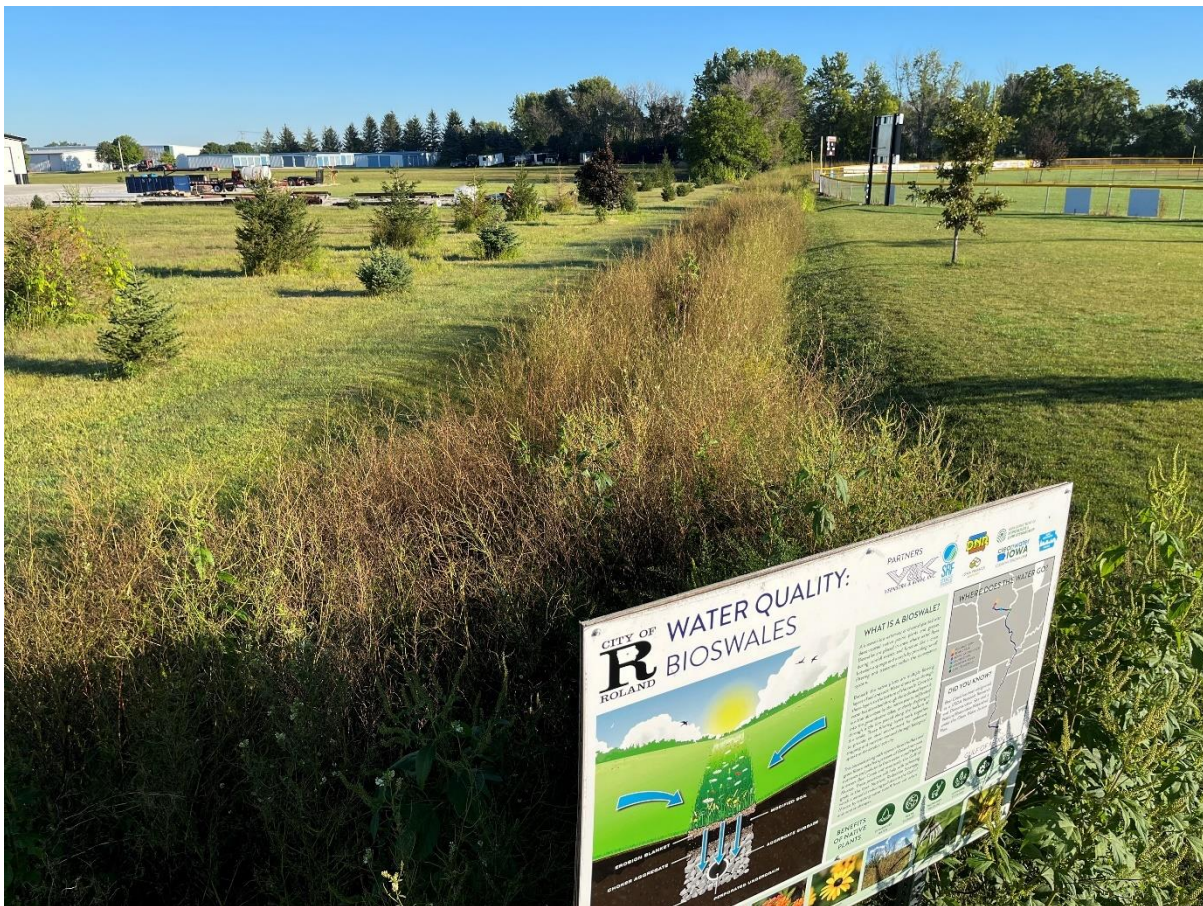
Figure 51: Bioswale Project in Roland Designed to Treat Urban Stormwater Runoff
